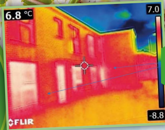
An example of the results from a thermal imaging survey
